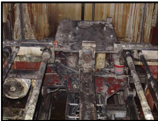
“Single-use” lubricators servicing pump bearings.
